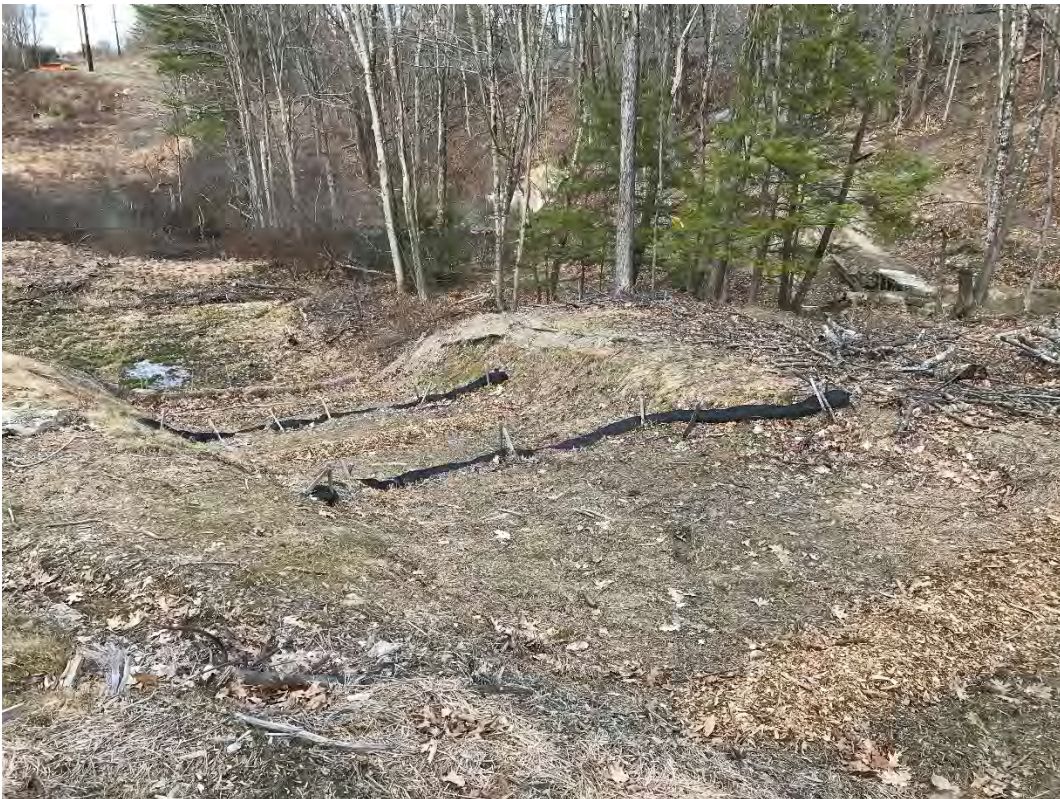
Fig 8: Lower portion of slope between Strs. 28 and 29. Viewing northeast. (04-06-21)
