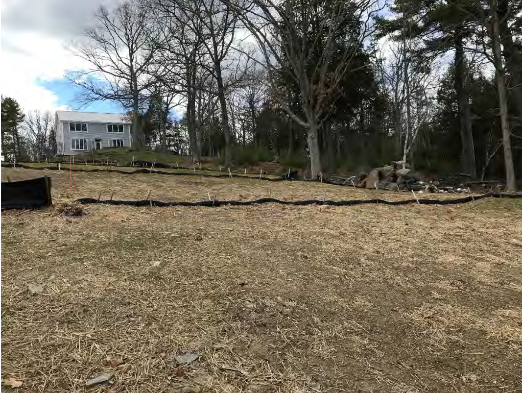
Fig 3: Slope above the cable house at the Eversource property/west side of the bay. Viewing northwest. (04-06-21)
