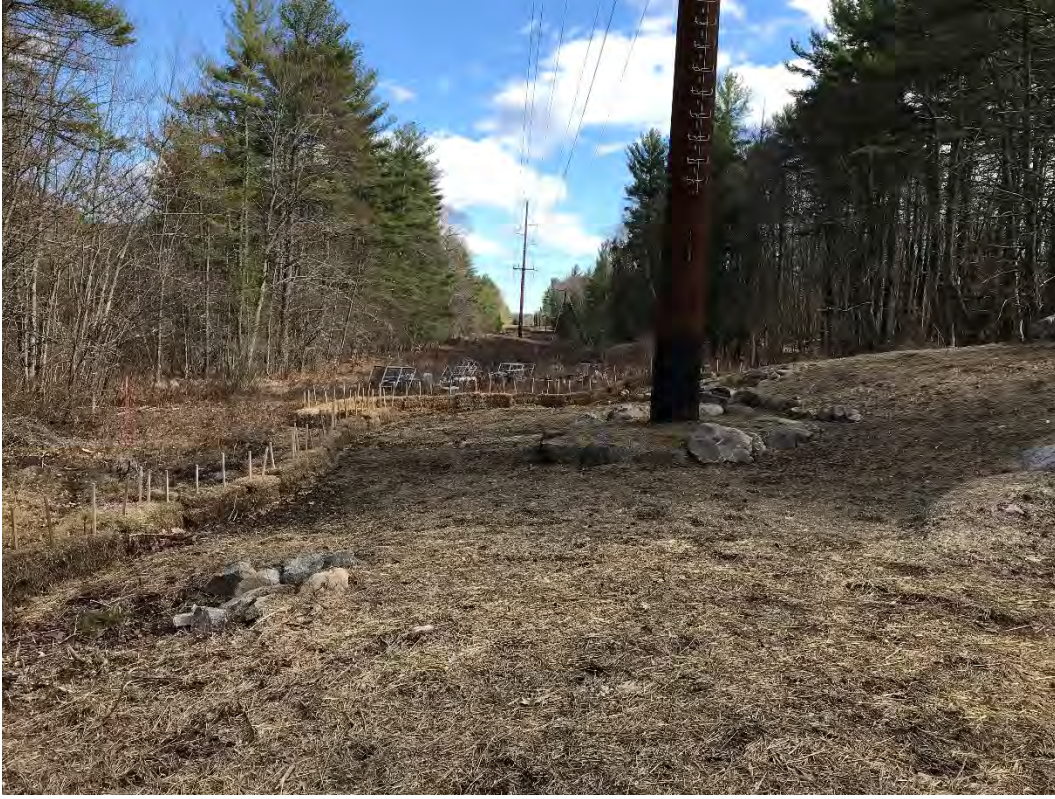
Fig 5: Str. 89 work area. Viewing southeast. (04-06-21)
