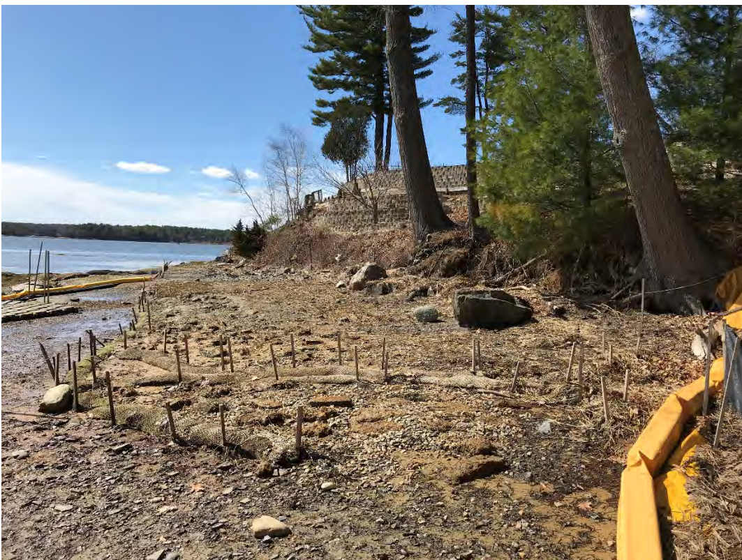
Fig 12: Salt marsh restoration at Gundalow Landing/east side of the bay. Viewing south. (04-06-21)
